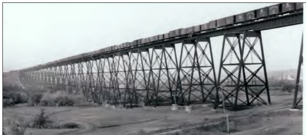
Railroad trestle crossing the Sheyenne River at Valley City
