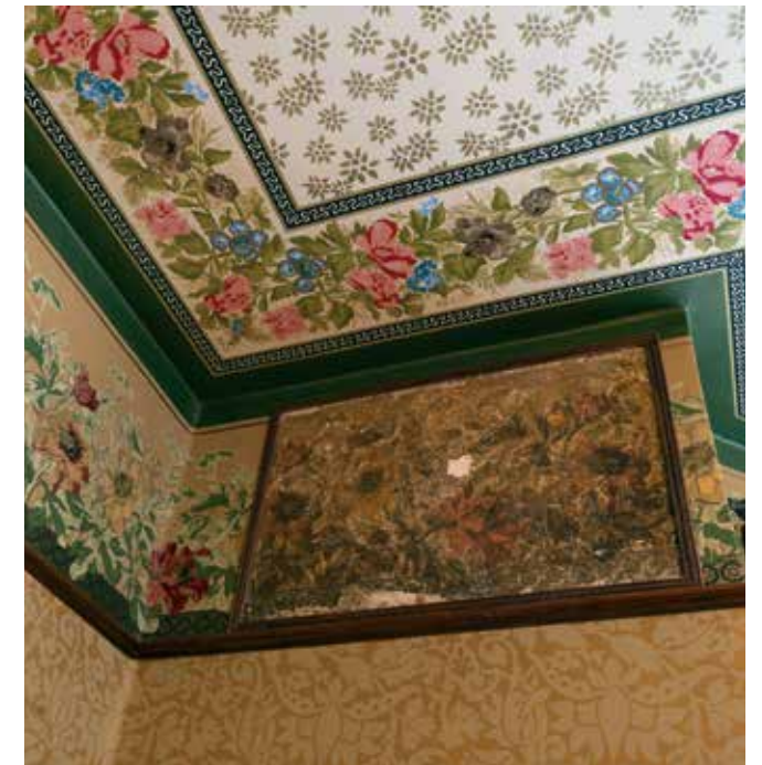
Corner of the Former Governors' Mansion parlor showing reproductions of the five different 1884 wallpapers. A framed section preserves an example of the original paper.
